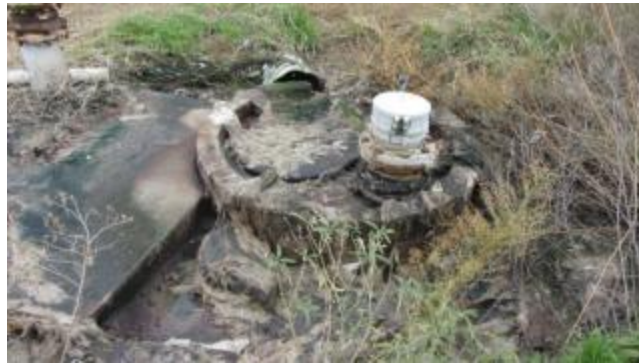
Sewage and rags around the Peridot Lift Station manhole. Culvert that transfers the wastewater into the wash downgradient of the lift station.
