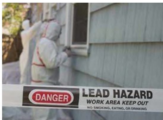
Image shows lead abatement work.
