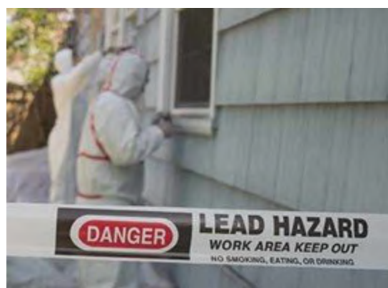
Image shows lead abatement work.
